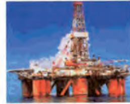
For distinguishing of drilling platform
